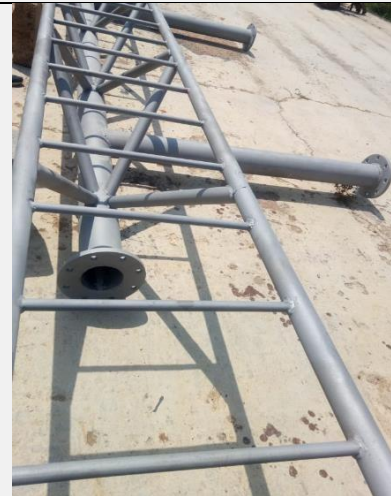
Pictures after abrasive blasting
