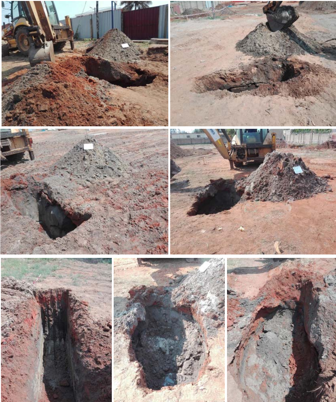
Figure 2.2 – Aspects of the trial pits implementation.
