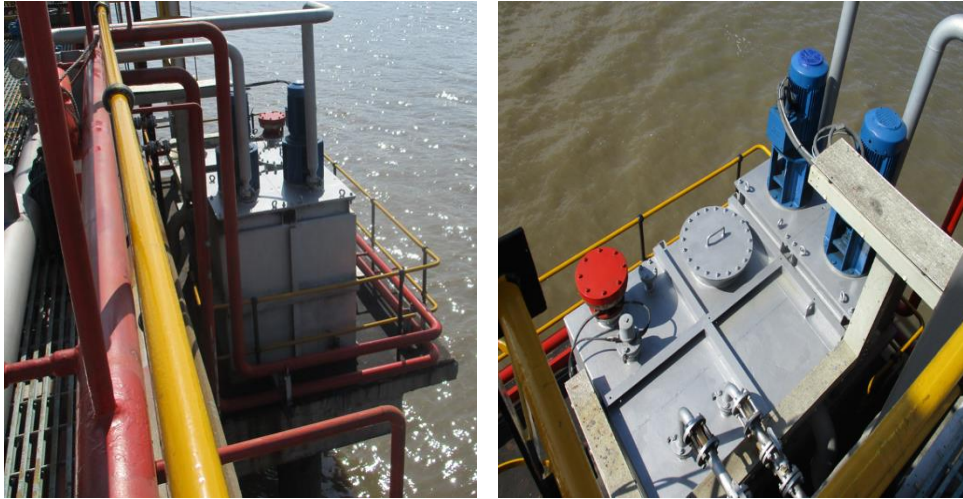
Figura 3.14: Tanque slop .
